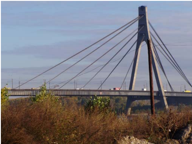
Cable Stayed Bridge, Kiev, Ukraine
